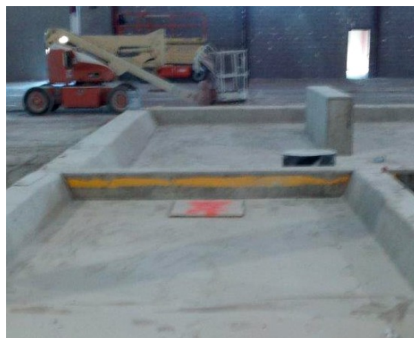
Appearance of RibLok after form removal.
