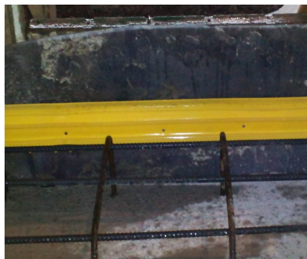
RibLok properly mounted on form. (Top row of screws hidden from view.)
