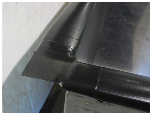
Fabricated top corner secured with Wittclips™.
