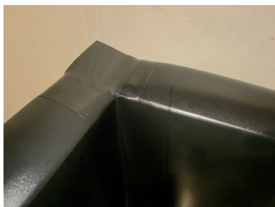
Perfectly formed corner with creases
